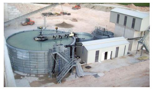
The water clarifying plant has the function to recover the dirty waters resulting from the washing of aggregates, in order to reuse them in the productive process. The principle of the functioning of our system based is on the clarification of dirty
